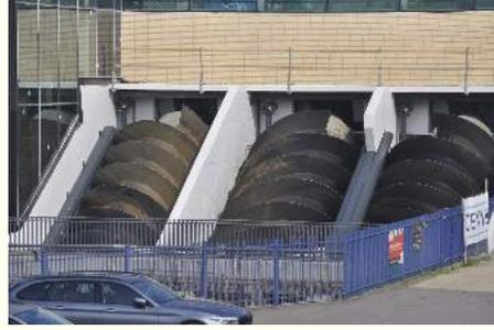
**A windmill in Kinderdijk with no wind blowing and a electric power driven Archimedean screw for removing water.**
