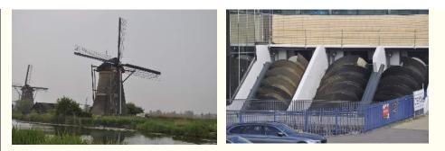
A windmill in Kinderdijk with no wind blowing and a electric power driven Archimedean screw for removing water.
