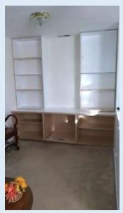
inch. After sorting that out, I cut the middle stiles first to final length, allowing ¾ inch below the cabinet for the inset doors to close on. The end stiles are cut to final length and somewhat over width for tapering to the walls on each end. Joined by glue and pocket screws, installed with glue and nails, bottom cabinets are almost complete. Face trim on bookcases are fairly easy, (assembled as the face trim on base cabinets) but also contoured to the wall on each side.
