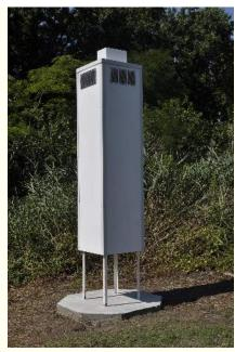
Installation of the vents and Hardie-Plank siding (Left) Finished product (Right)
